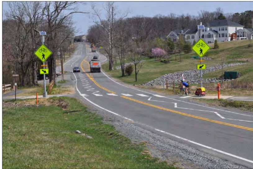
Figure 5. RRFBs and Signage at W&OD Trail Crossing
