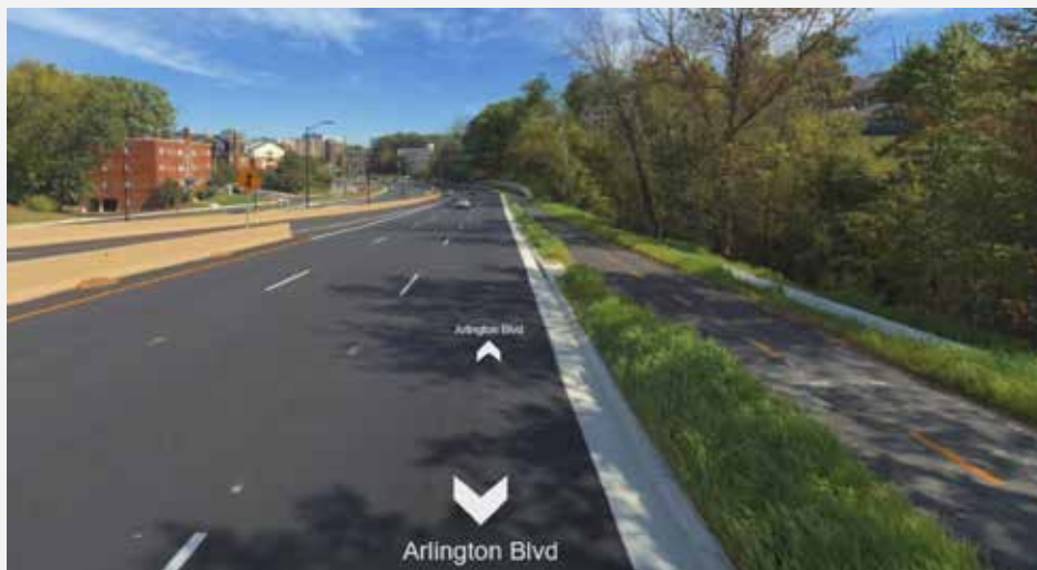
Figure 15: Arlington Boulevard in Arlington County. Arlington Boulevard (US 50) near Courthouse Road is an example of a Multimodal Through Corridor that accommodates all travel modes, including bicyclists and pedestrians with shared-use paths on both sides of the road (Image Credit: Bing Maps)
