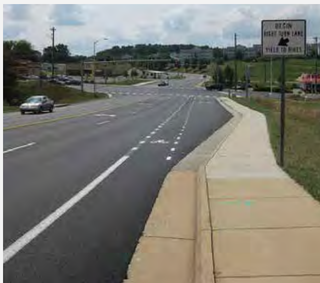
Figure 87: Bicycle Lane Transition at Intersection. Dashed lines indicate motor vehicles may encroach into the bicycle lane to enter the right turn lane and warn drivers to yield to bicyclists. Image source: City of Harrisonburg.
