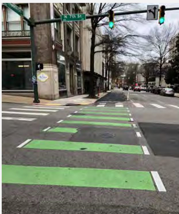
Figure 88: Green Dashed Pavement Markings for Bicycle Lanes Through Intersections. At the intersection of East Franklin Street and North 7th Street in Richmond, green paint supplements the white dashed lines indicating the continuation of the bicycle lane through the intersection. (Image Credit: EPR, P.C.)
