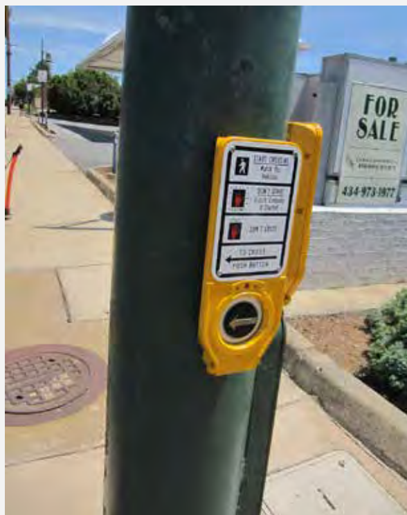
Figure 82: Activated APS Push-Button. This traffic signal is activated, meaning pedestrians push the black button to call a pedestrian phase to cross the street. It is also an APS that speaks the name of the street and vibrates when the pedestrian phase is on.
